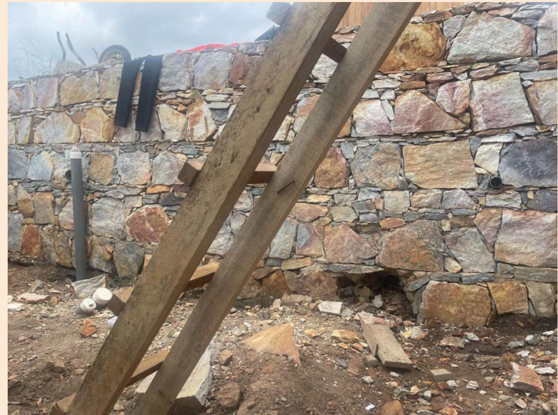
Water tanks and underground septic system
