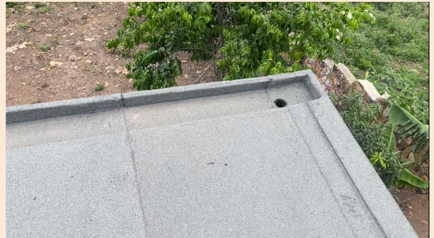
(Roof with gutter and pipes)
